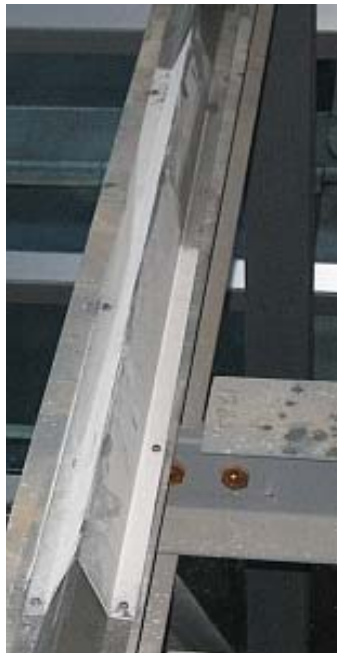
Beveled ledge in hoistway
