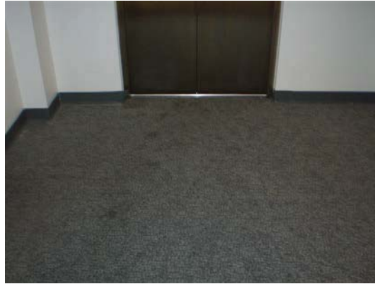
Elevator lobby flooring
