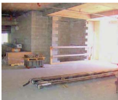
Access for delivery of material
