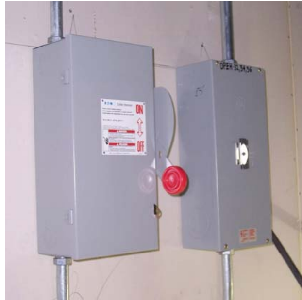
Three-phase disconnects shown on left; car lighting disconnects shown on right
