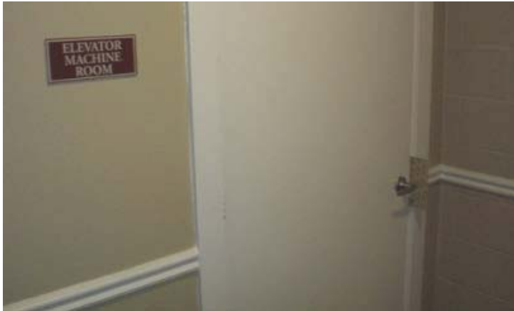
Self-closing, self-locking machine room door
