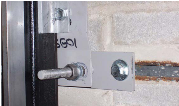
Insert with bracket and rail attached
