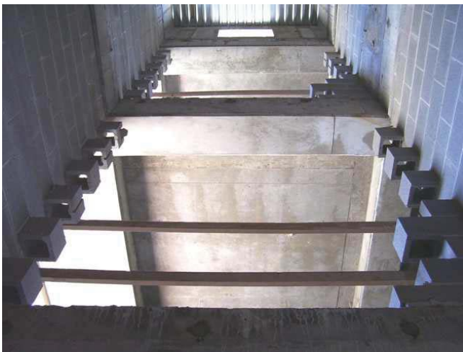
Front wall open before installation of equipment, block wall construction
