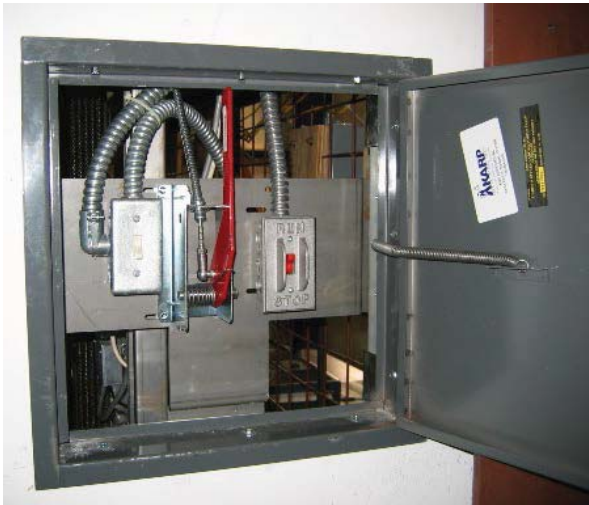
Manual brake release access panel
