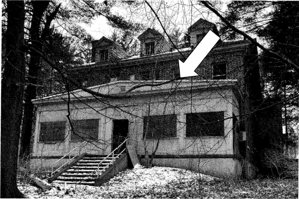
Roofing - Front Porch Roof
